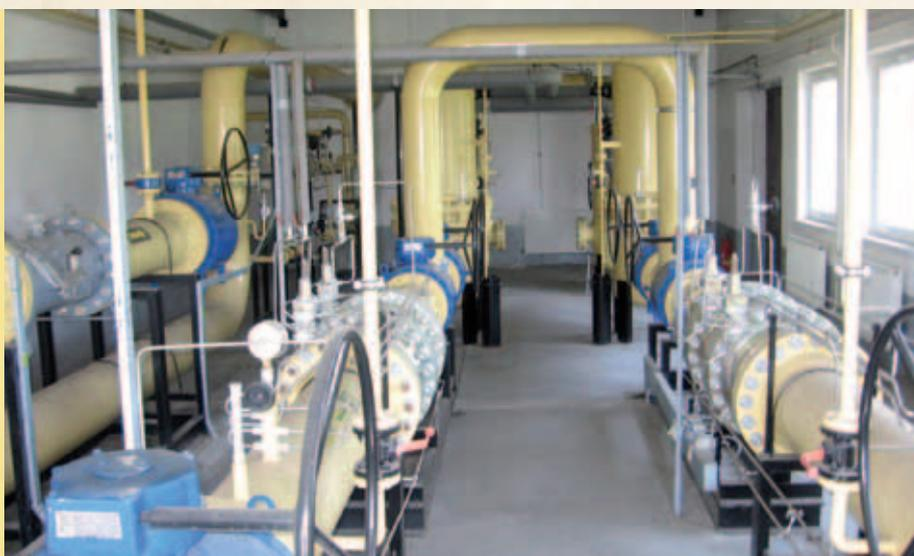
Technological equipment of the Delivery Station in Záhorská Bystrica - significant technological object regulating the level of gas pressure from 4.0 Pa to 2.5 MPa for the Bratislava area
