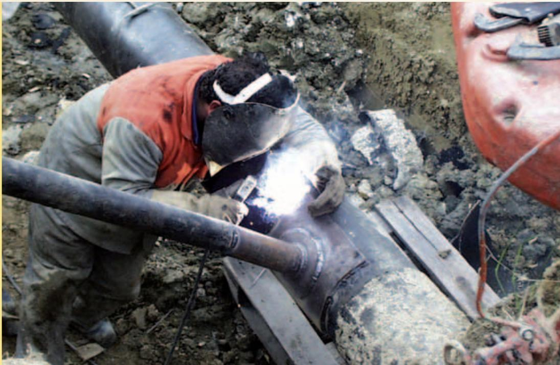
Surfacing of the bypass pipeline of the route valve near the village Jamnik
