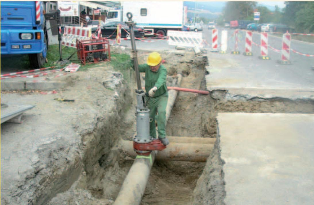
Pipeline closing on medium - pressure pipeline during reconstruction works
