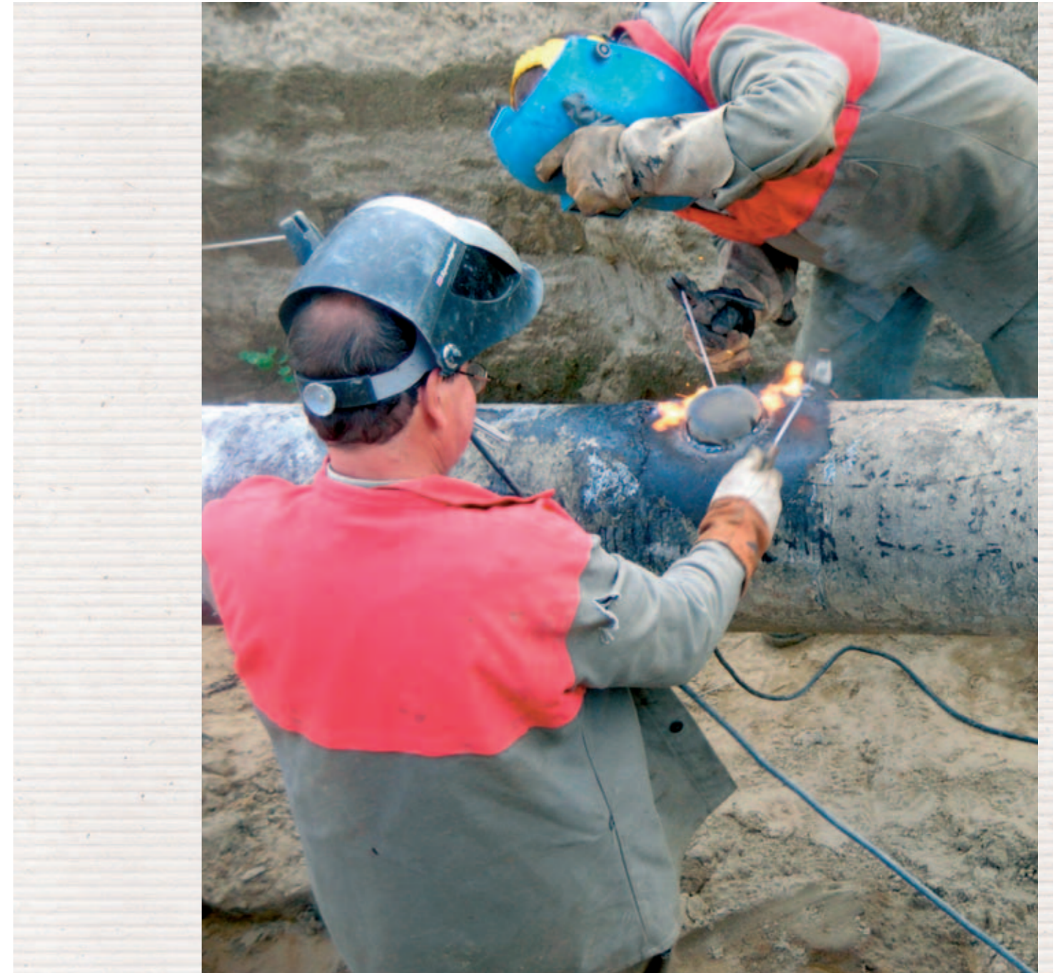
Welding on high-pressure pipeline during reconstruction works
