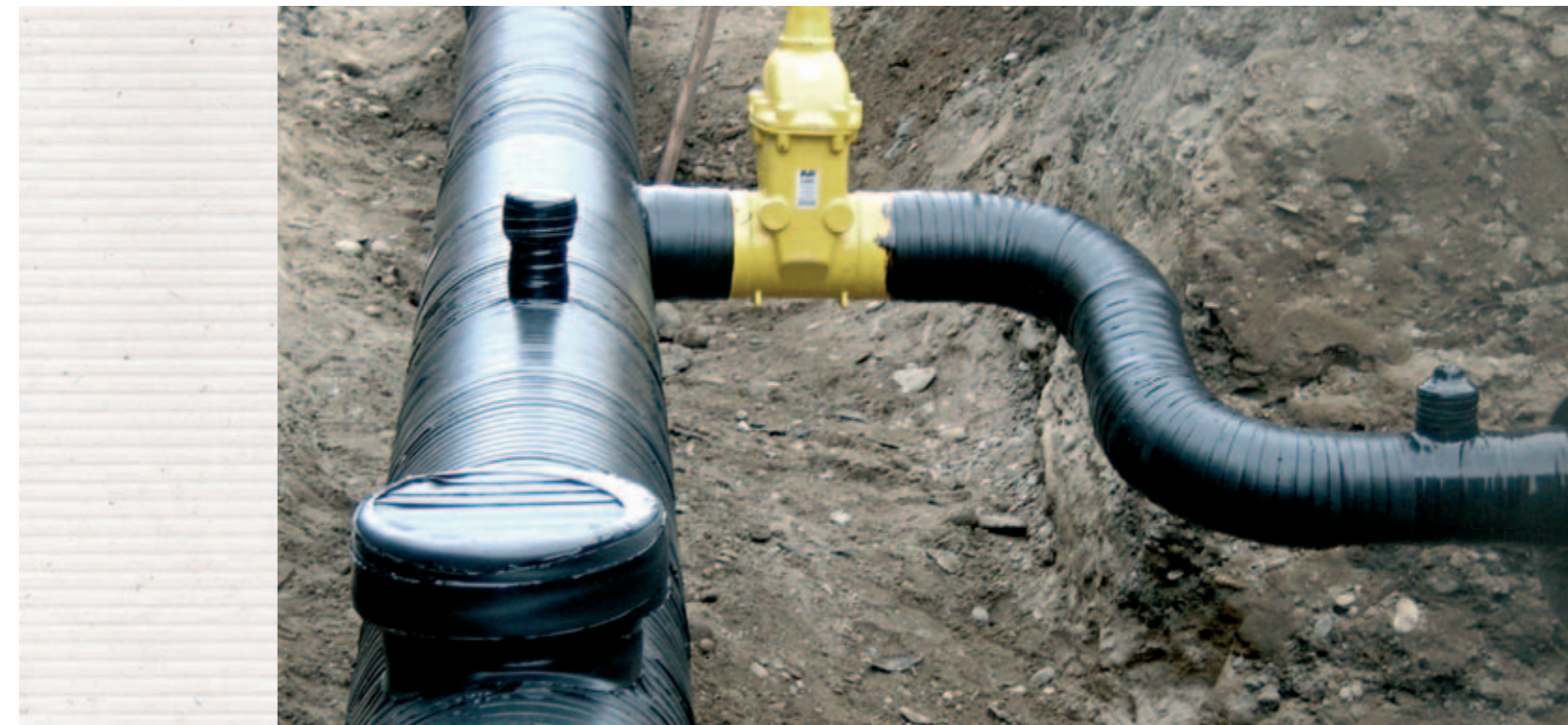
Reconstructed pipeline before completing the surface finish
