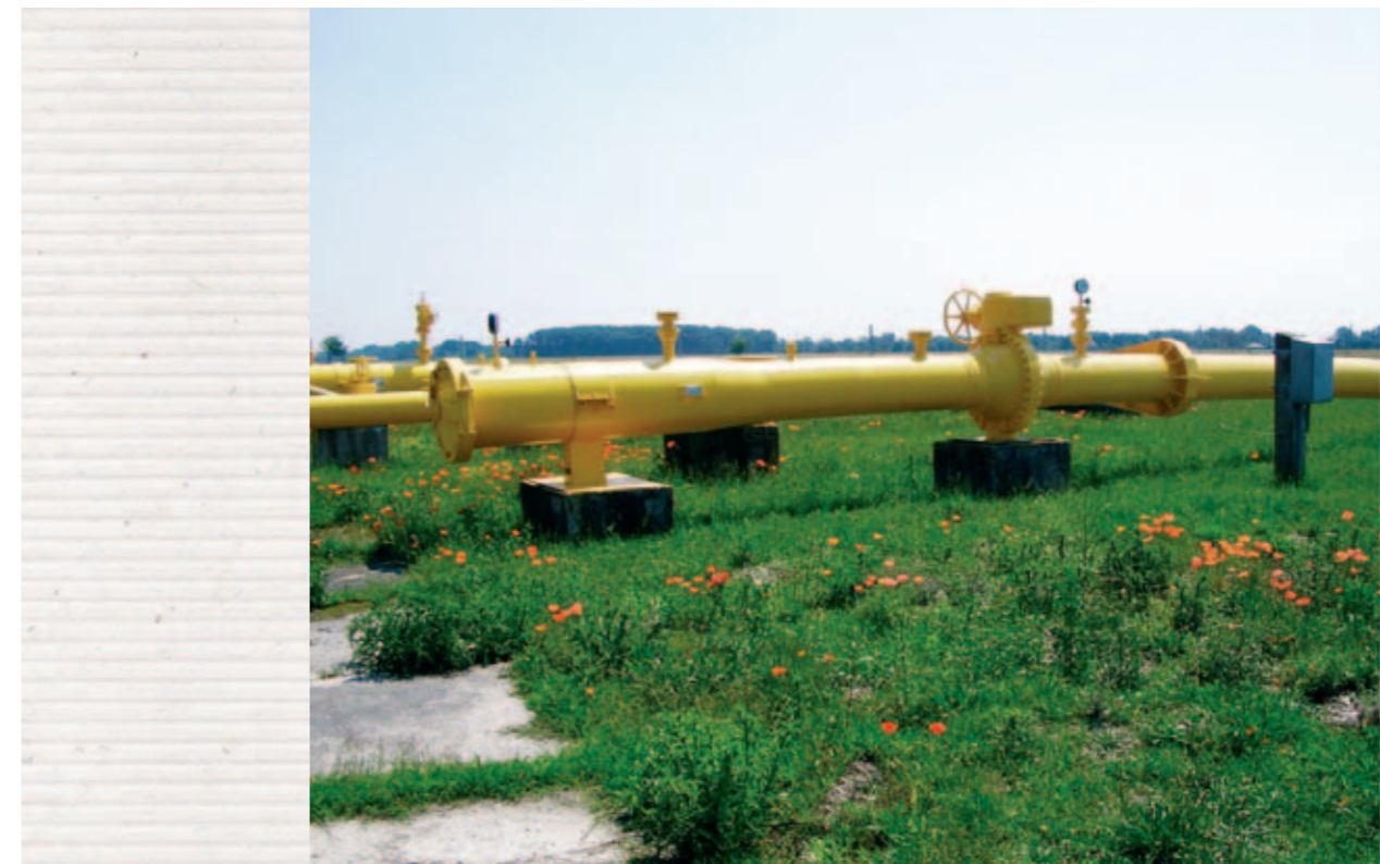
Launcher for the insertion of cleaning and monitoring device, so-called pig, to the high-pressure gas pipeline
