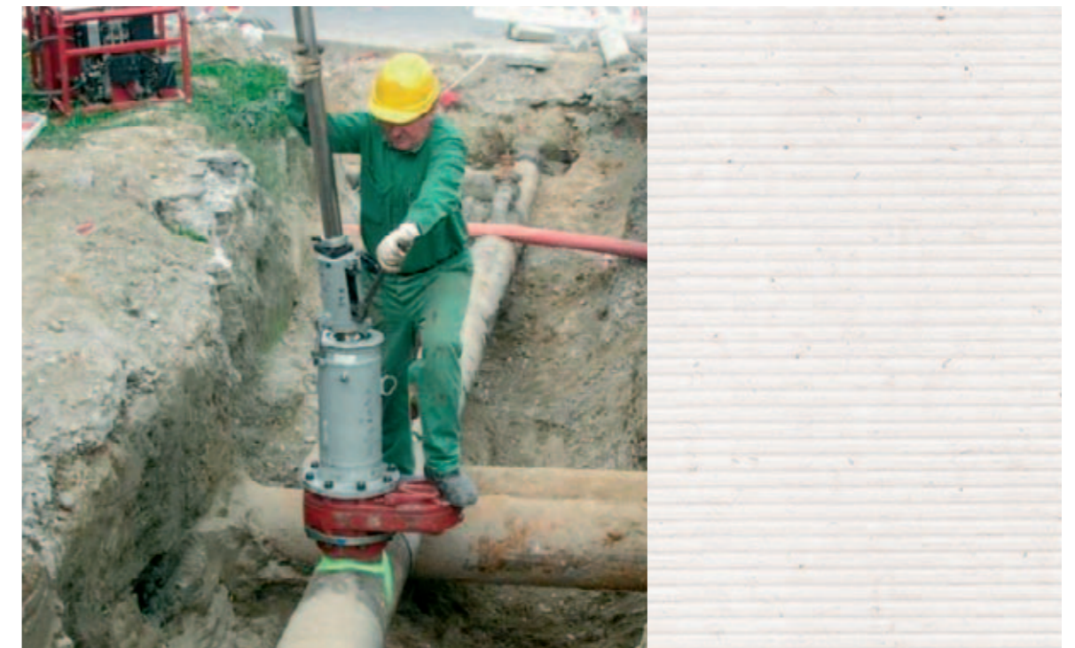
Pipeline closing on medium-pressure pipeline during reconstruction works
